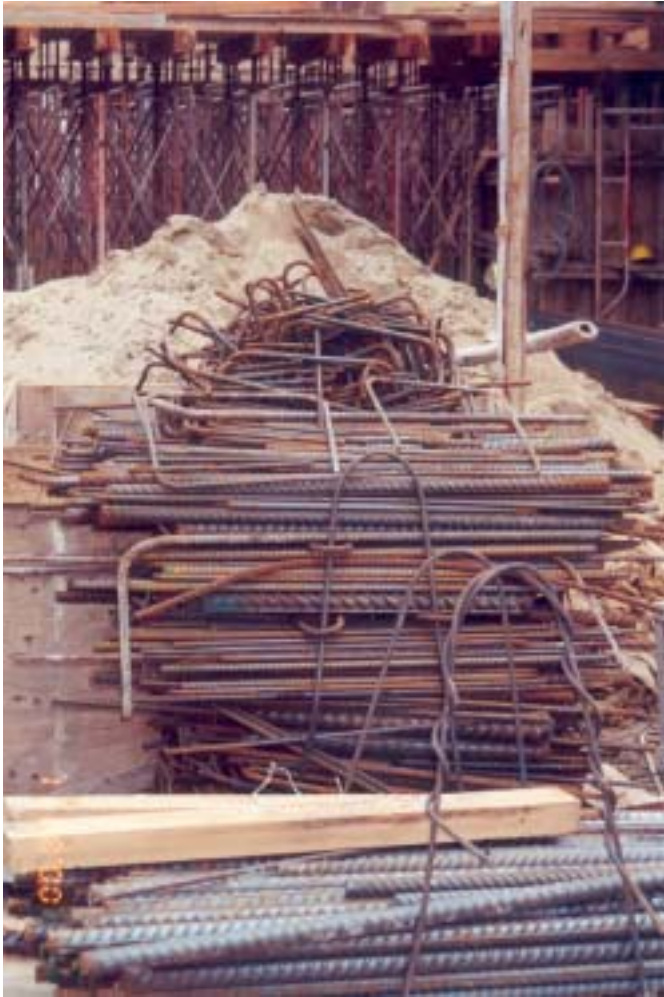
Left page: sorted reinforcement bars cutting waste, to be recycled. Right page: Unsorted construction waste.
