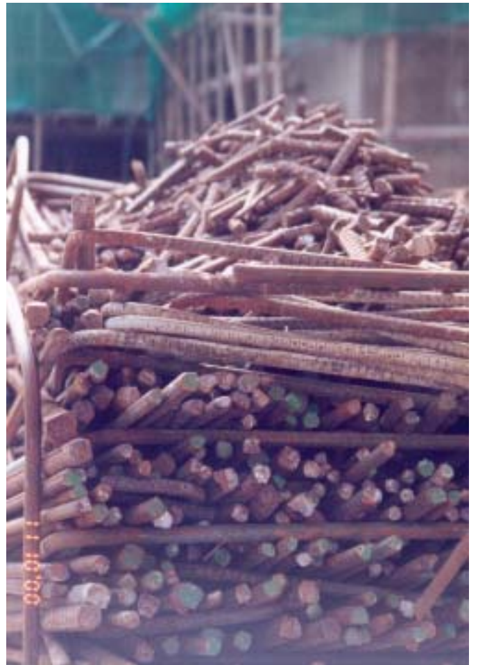
Left page: sorted reinforcement bars cutting waste, to be recycled. Right page: Unsorted construction waste.
