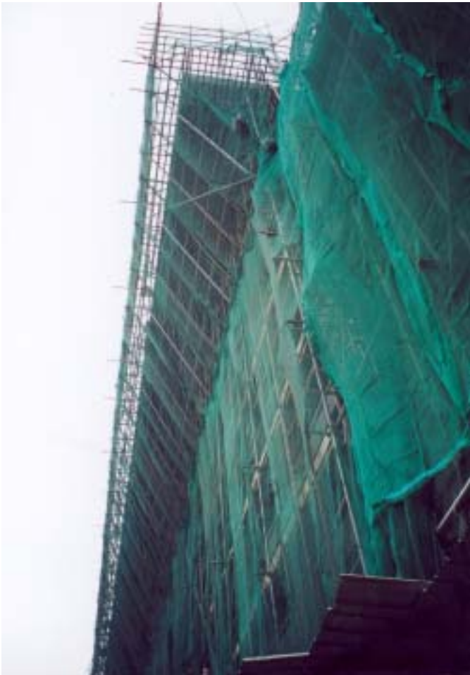
Top: Metal scaffolding. Bottom: Mixed bamboo and metal scaffolding.
