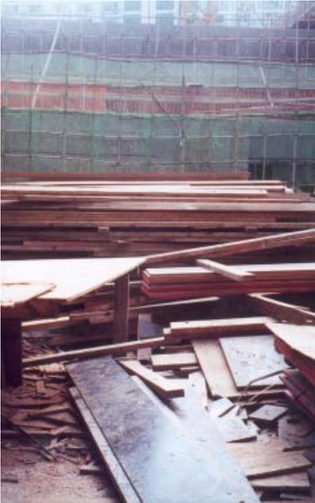
Left, Timber cutting formwork. Right, Tiling waste from cutting.
