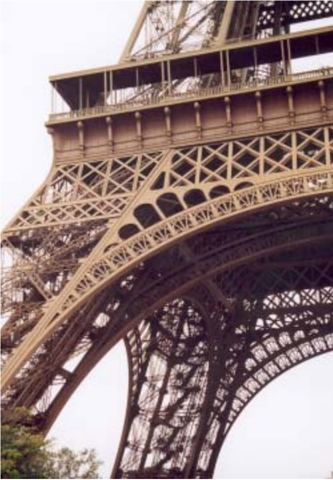
Left page: The steel structure of the Eiffel tower can be dismantled as it was designed as a temporary building for exhibition, Paris, France. Right page: Mongolian yurt, 18th century (Source: Detail serie 6, 2000).
