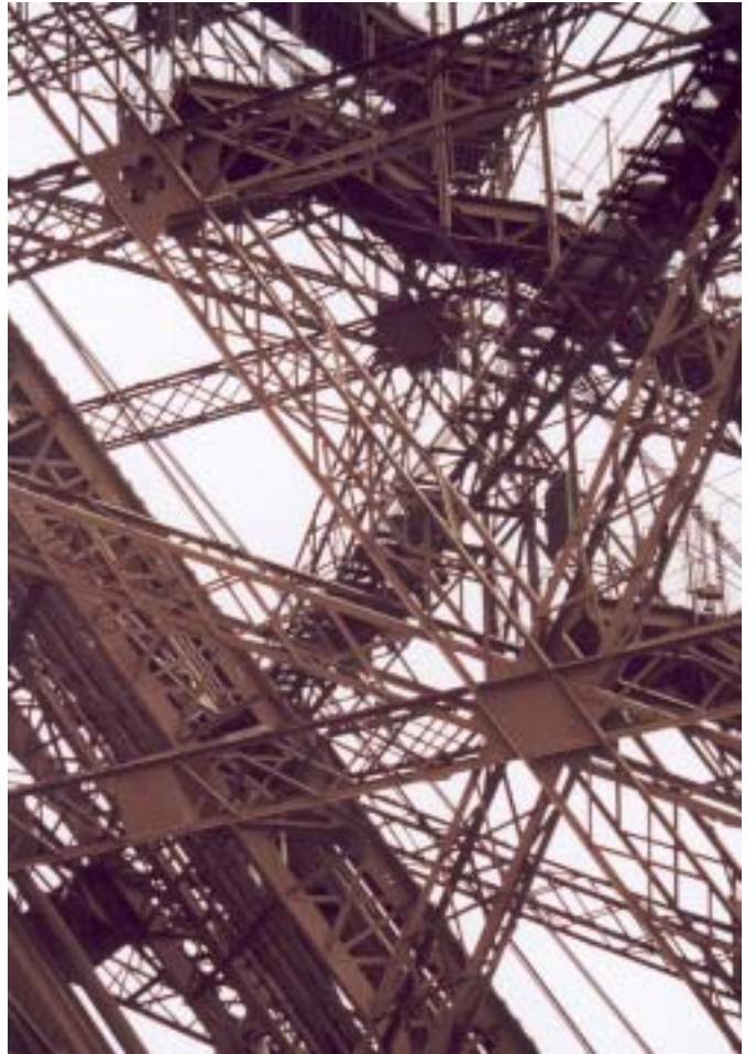
Left page: The steel structure of the Eiffel tower can be dismantled as it was designed as a temporary building for exhibition, Paris, France. Right page: Mongolian yurt, 18th century (Source: Detail serie 6, 2000).
