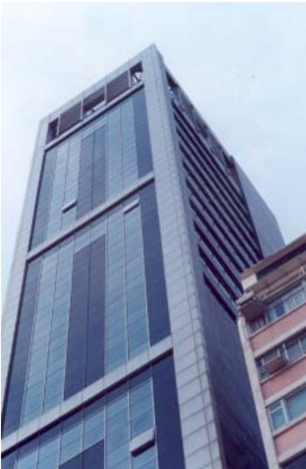
Views of the external renovation. The original building is the brown part of the building. A new skin has been added to the original facade.
