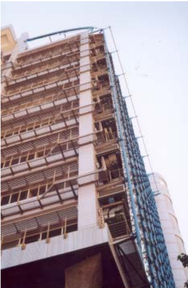
Right page: Kadoorie Biological Sciences building second skin system facades, section and typical laboratory floor plan (source: Building Journal Hong Kong China, May 2000, Kadoorie Biological Sciences Building, Beneath the Second Skin , Tam Angela).
