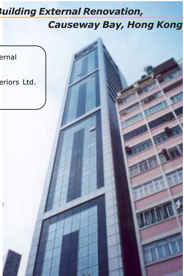
Views of the external renovation. The original building is the brown part of the building. A new skin has been added to the original facade.
