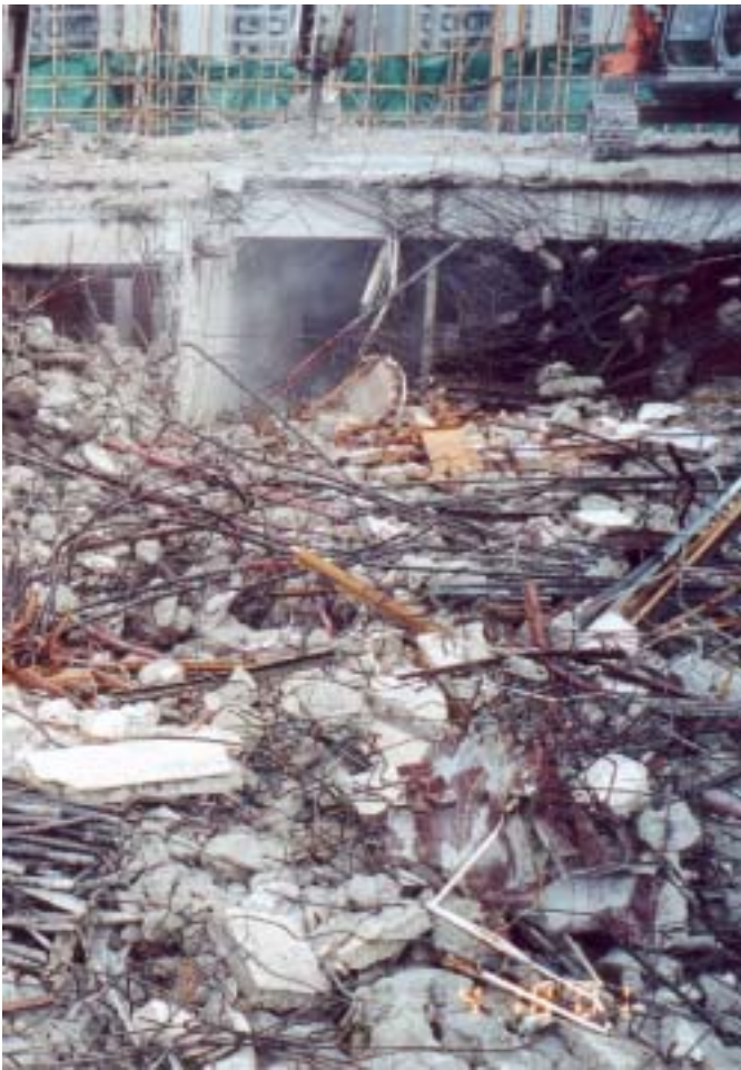
Mixed demolition waste
